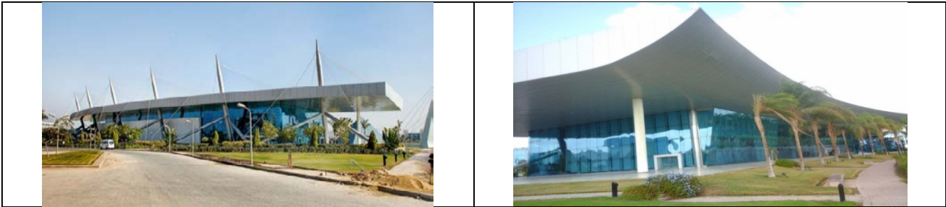
Fig. 8 External view of the conference center (Smart Villages 2015)
